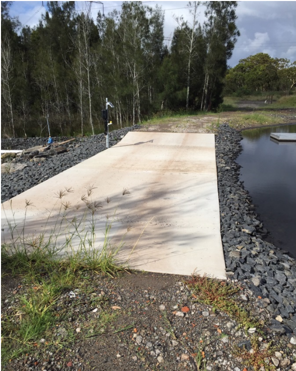
Photo 2. Installation of an engineered two stage spillway, for low (typical flow rates) and high flow rates.
