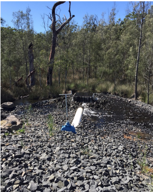
Photo 3. Installation of an engineered discharge point
