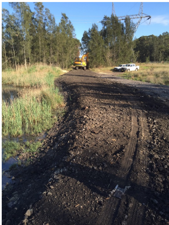
Photo 1. Repairs and raising of Dam 10 embankment.
