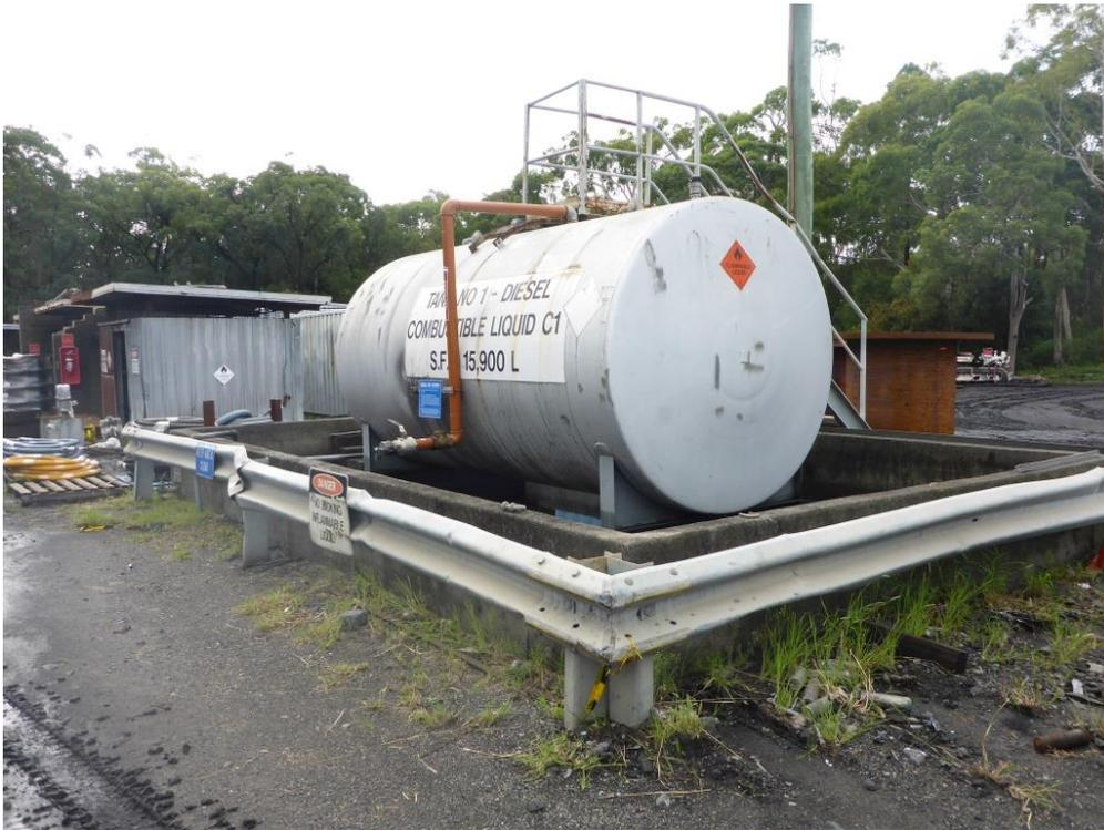
**Photo 5 Diesel Tank stored within Bund**
