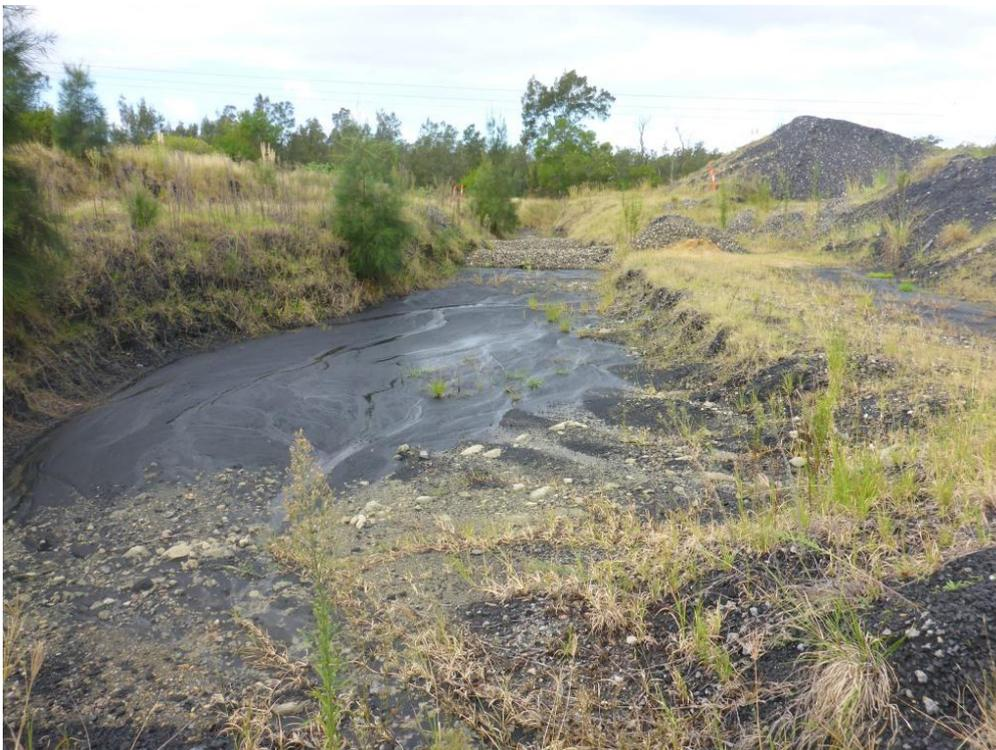
**Photo 6 Coal Material in drain should be removed**
